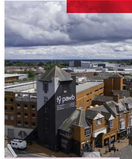
Ty Pawb, Wrexham, North East Wales Credit: Crown Copyright
