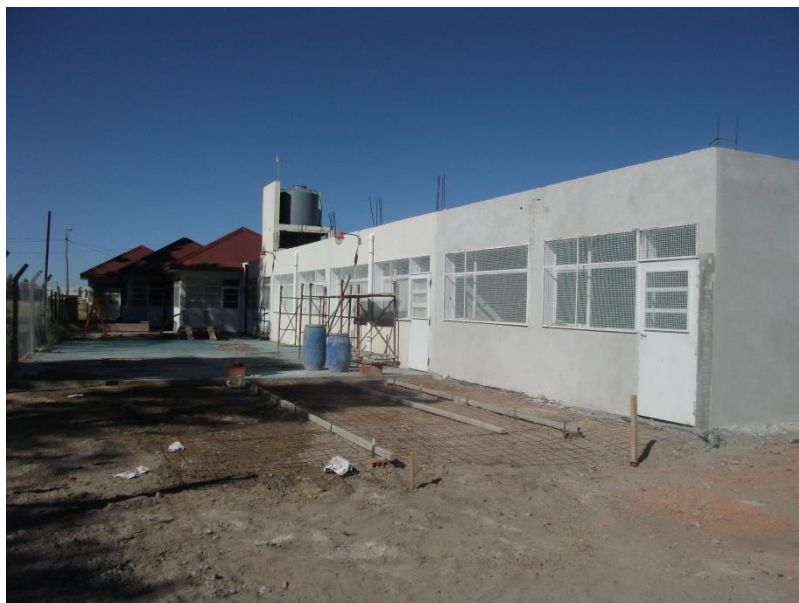
The building work for the new classrooms at Ysgol yr Hendre
