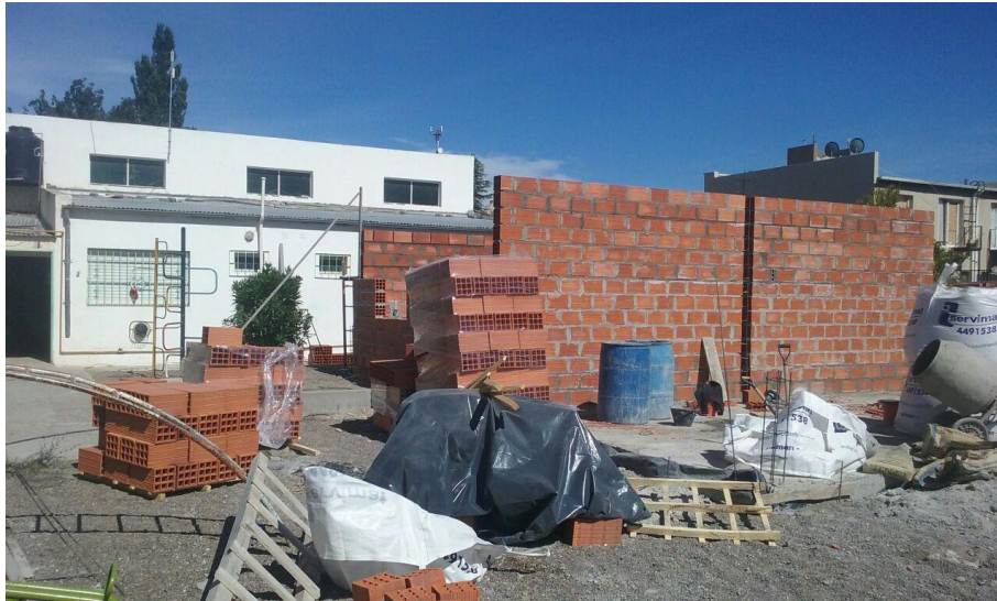
Building two new classrooms at Ysgol Gymraeg y Gaiman
